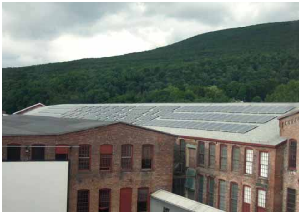
Figure 3: The 50 kW installation at Mass MoCA. Photo courtesy of Ruth Aronoff.
