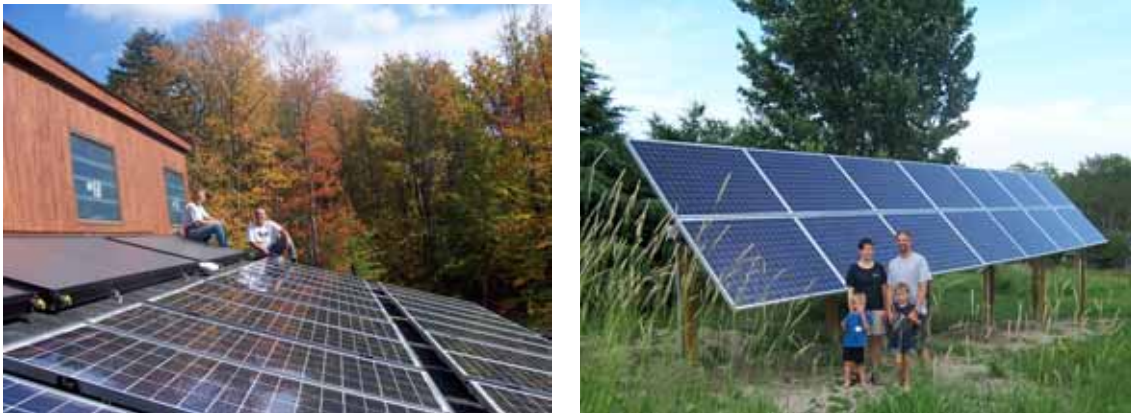
Figure 1: At left, a roof-mounted array on a south-facing roof on a house in Becket, MA. At right, a pole-mounted array. Photos courtesy of BPVS 1 .
