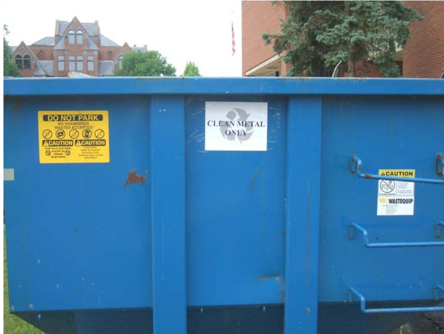
Figure 7. Example of on-site sorting of recyclable C&D waste. Allied Waste designates dumpsters for different types of waste.
