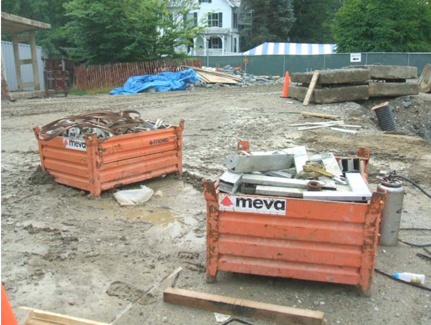
Figure 5. Additional examples of both scrap materials and packaging waste from the North and South Academic Buildings construction site.
